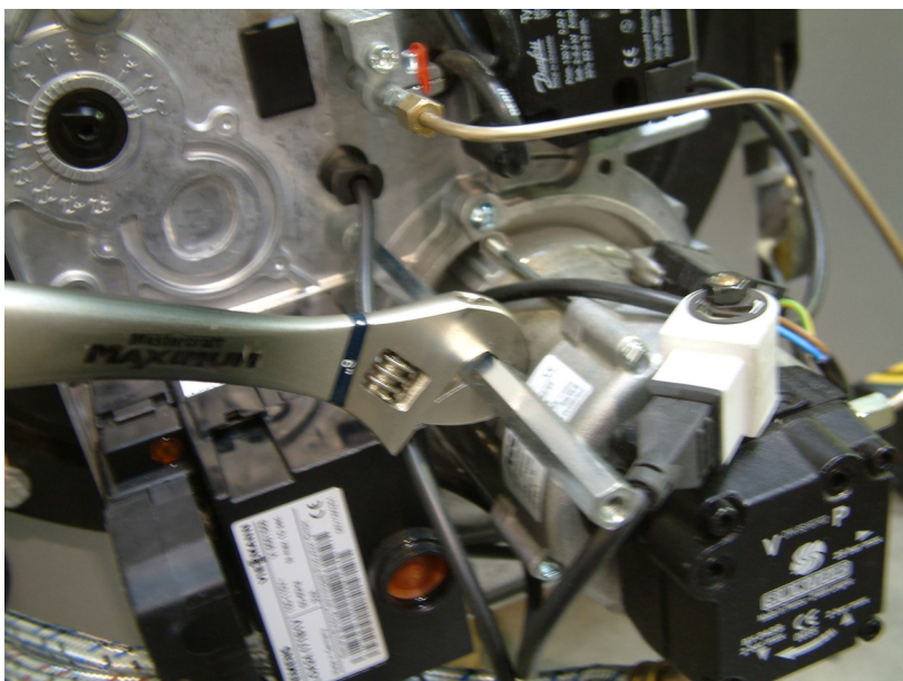
Fig. 12 Tighten the extension bolt.
