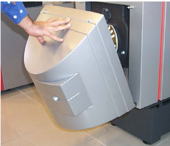
Fig. 7 Mounting the burner hood
